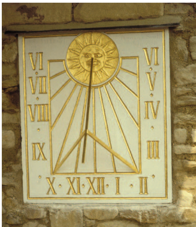
Fig. 3. An example of a completely reconstructed "17th century" direct vertical sundial on the Martin Tower in the Tower of London, designed by the author and carved by Messrs Plowden & Smith in 1988. The face of the original dial-plate had suffered from severe weathering and had been entirely worn away, whilst the metal gnomon had survived until c. 1938. A new dial-plate of Portland stone was affixed over the original stone-work, incised with a 17th century design. (Clocks Magazine, 'The Sundial Page', p. 20, Vol 23/2, March 2000)
