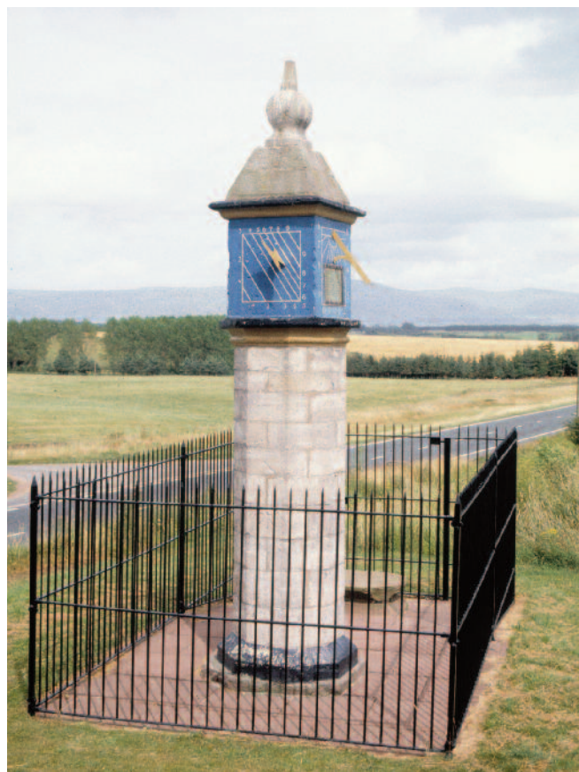
Fig. 4. An example of a restored pillar dial – the Countess's Pillar, erected by Lady Anne Clifford in 1656 at Penrith in Cumbria – with an element of reconstruction design by the author, in the provision of a new gnomon for the south face. The dial was restored (repainted) by English Heritage in 1984-85. (Clocks Magazine, 'The Sundial Page', p.35, Vol 20/9, September 1997)
